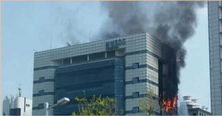
Major fire at a Samsung data center in Gwacheon, South Korea, 2014
